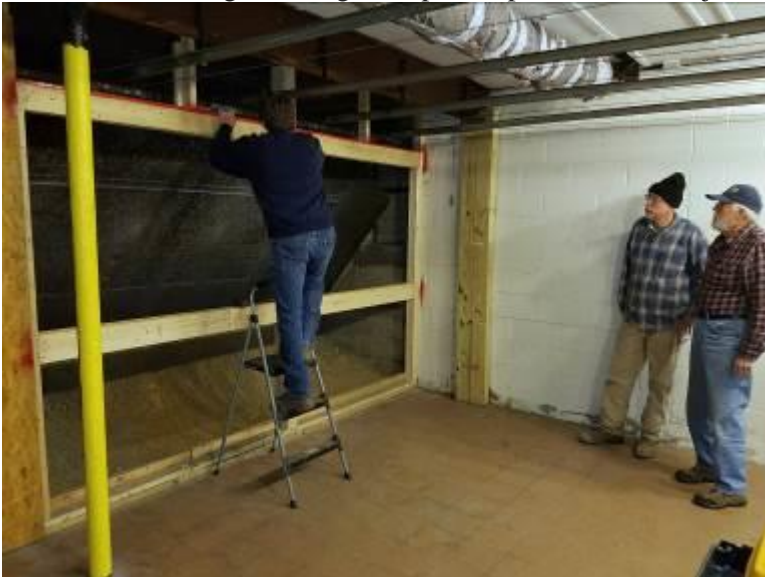
Jim Coach finishing screwing head post in place - one-man job!
