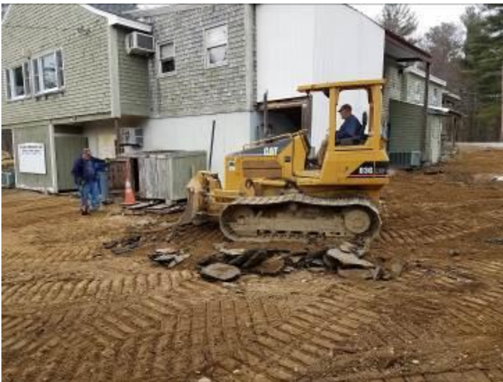
Front Parking Lot Graded
